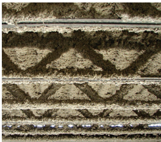
Figure C-4: Fireproofing added to structural steel
