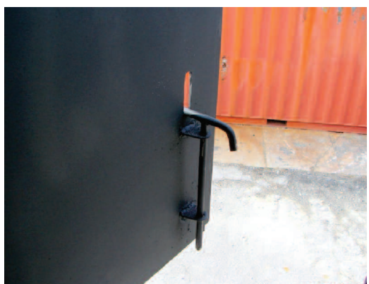
Figure C-6: Window & Latch Construction
